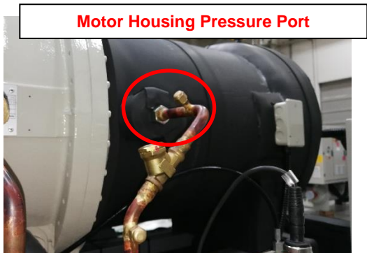
Detail of motor housing. Possibility of residual pressure in this part.
