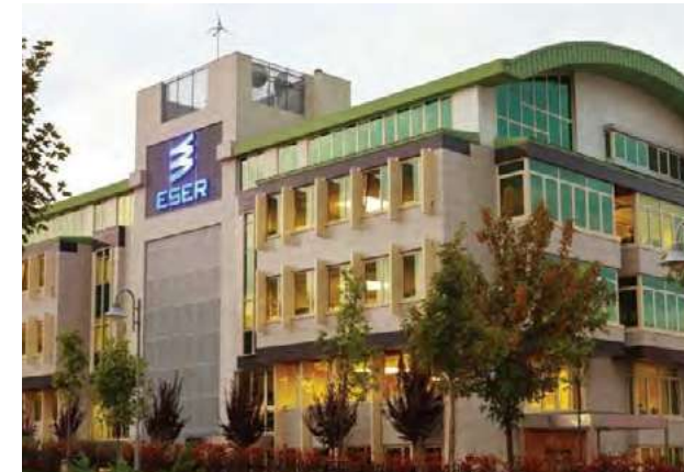
Eser Holding-LEED PLATINUM
