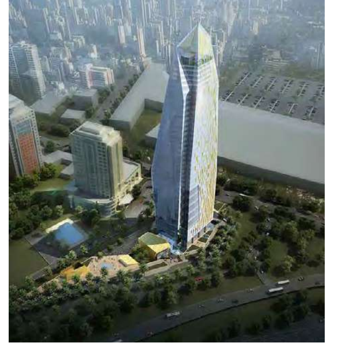
Rönesans Allianz Tower-LEED PLATINUM
